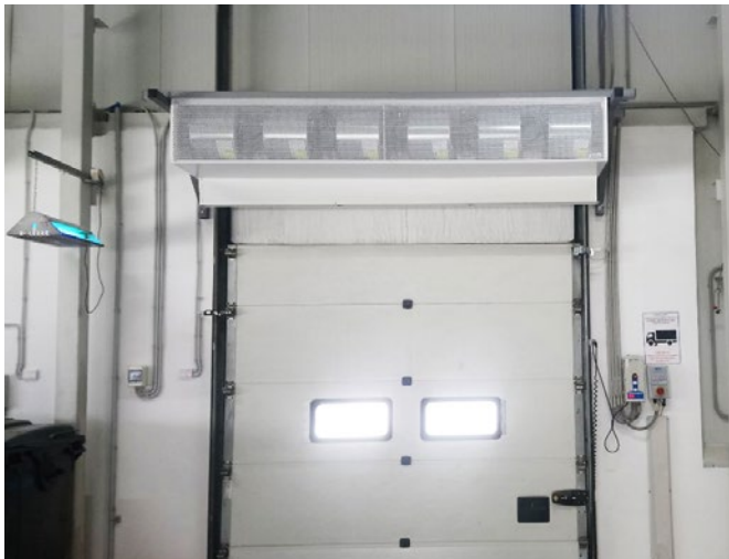
Fly KXL Installation in factory doorway
